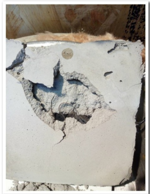
#24 Cement tile blown by heating with retained moisture - B
