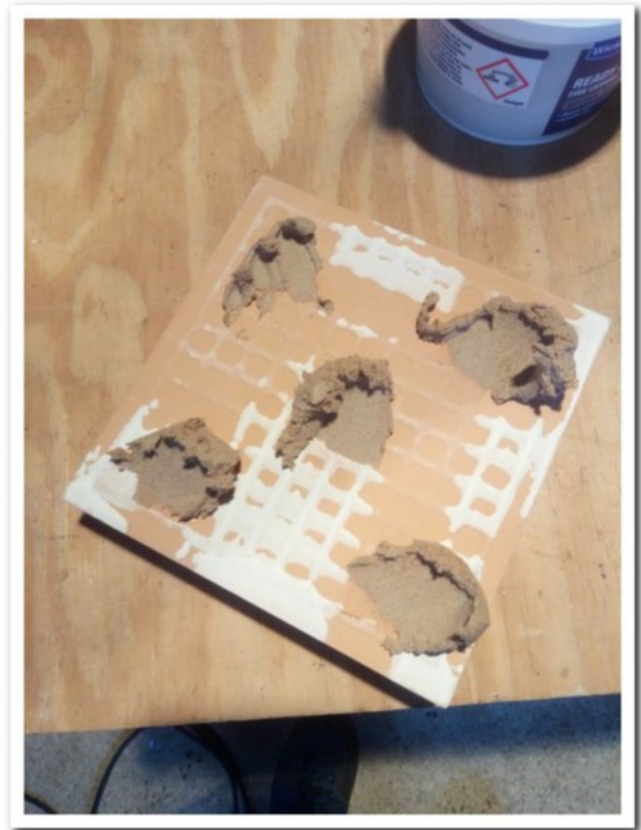
#10 Dabs of cement/mortar used as per wall tiling
