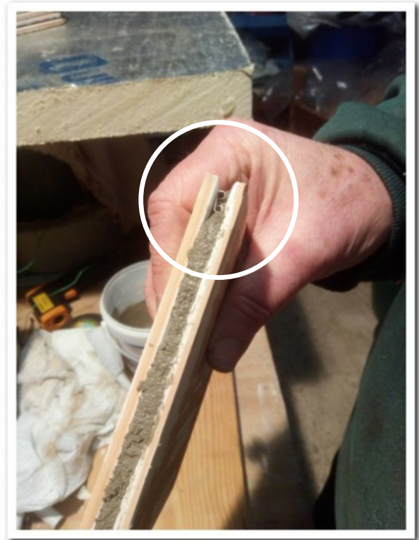
#22 Push fit connector being encased in cement
