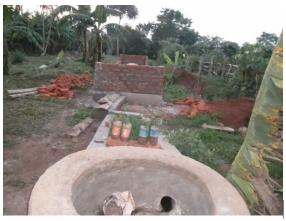
The mouth where cow dang is put and mixed with water was build on the Flexigester to enable better mix of dung with water.
