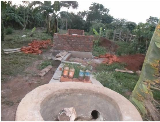
The mouth where cow dung is put and mixed with water was built on the Flexigester to enable better mix of dung with water.
