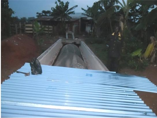
A tin roof was installed above for the same reasons above and to also increase on the heat needed by the Flexigester to produce more gas.
